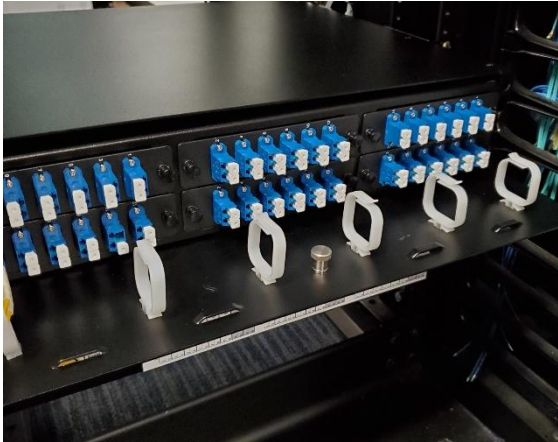
Figure 21: Cable routing rings inserted into specified holes in panel insert.
