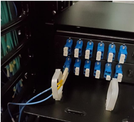
Figure 22: Cable routing rings managing patch connections and cover replaced.
