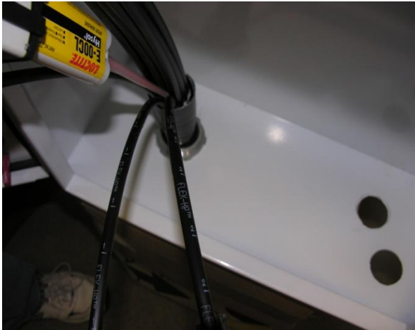
Figure 19 Epoxy Sealant Injected Between & Around All Tubes
