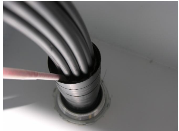
Figure 20a Injecting Epoxy Sealant in Open Space Between Outer Ring Tubes and Encapsulant Container
