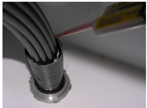
Figure 20b Completing the Epoxy Sealant Application
