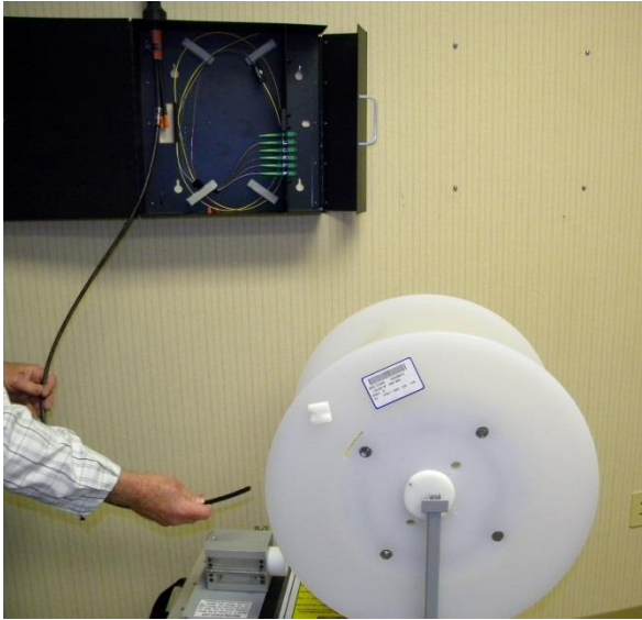
Figure 9 Ready Tubing and Empty Reel at Exit Point FTU
