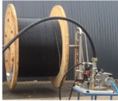
Fig. 2 Air-blown installation method
