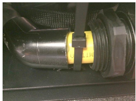
Figure 13 Tie Down Protruding From Patch Rear
