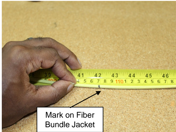
Figure 1 Marking Fiber Bundle Outer Foam Jacket Between 42" - 44" for 72 Fiber Bundles
