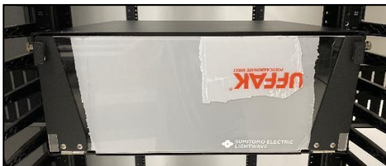
Panel Mounted to rack using large screws
