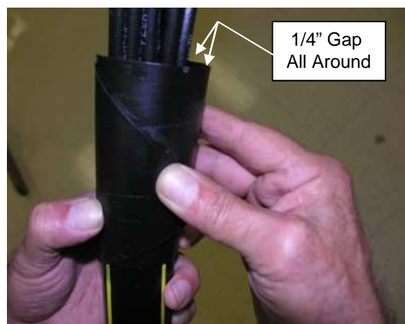
Figure 15 Final Positioning of Encapsulant Container Before Taping in Place
