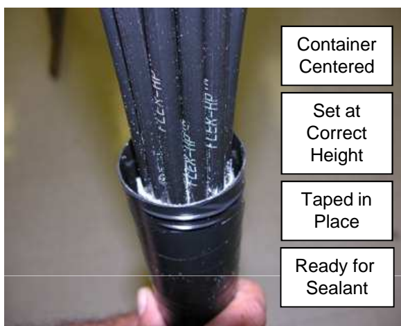
Figure 16 Encapsulant Container Installed Properly
