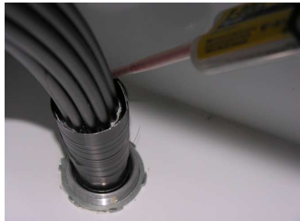
Figure 20b Completing the Epoxy Sealant Application
