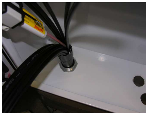
Figure 18 Injecting Epoxy Sealant Between & Around Next Tubes (Working Forward)
