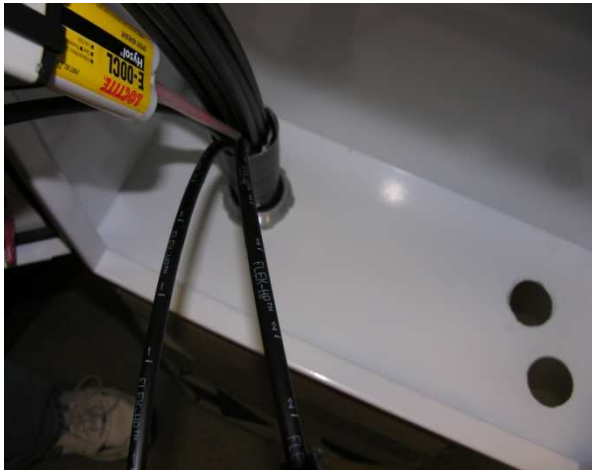
Figure 19 Epoxy Sealant Injected Between & Around All Tubes
